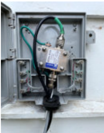
Figure 8 – Final Configuration of the Arrestor Box [16]
