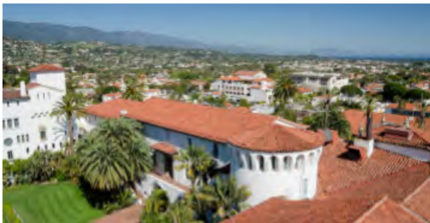
[Above] Mission Santa Barbara after the earthquake.
