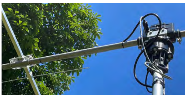
Figure 9 - Wooden Crossboom Replaced
